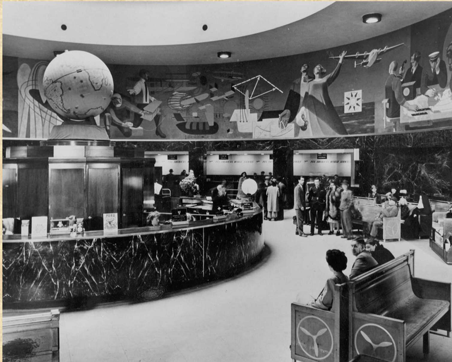
1940 An inside view of the Marine Air Terminal
