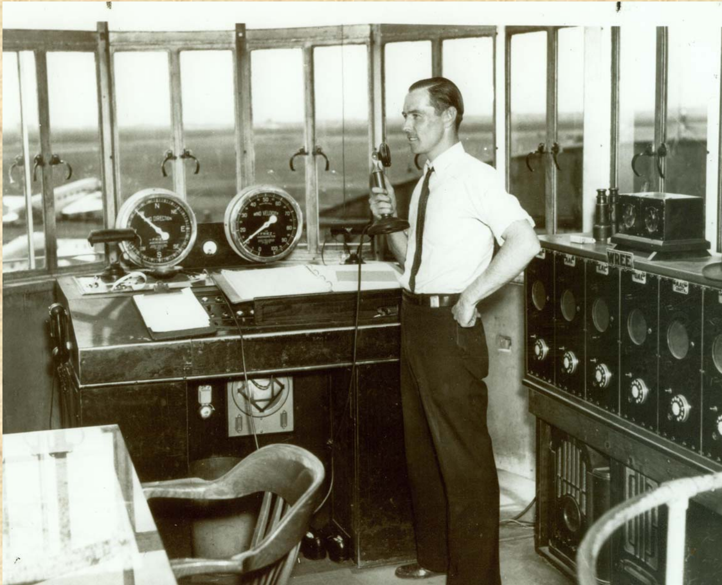
1936 The first radio equipped tower at the Newark, NJ, airport
