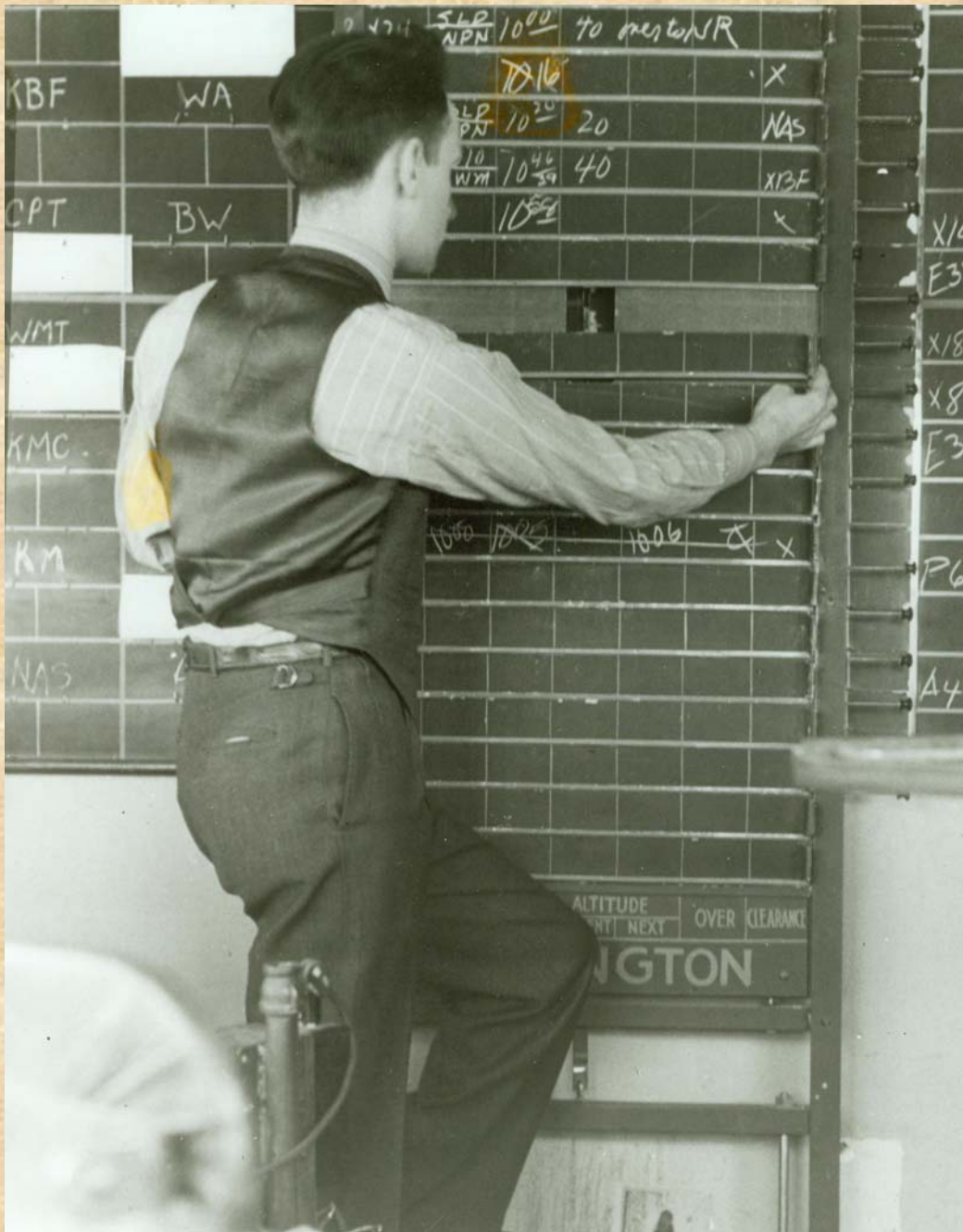
1940s The first effort to automate air traffic control using slats
